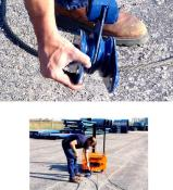
Pull the cable back to the front of the puller and attach it with the large shackle.
