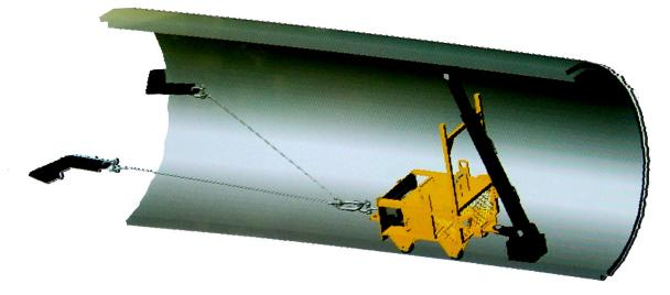
Once you have safely secured a position outside of the pipe, retract the cable until the new pipe begins to mate with the previous installed pipe.
