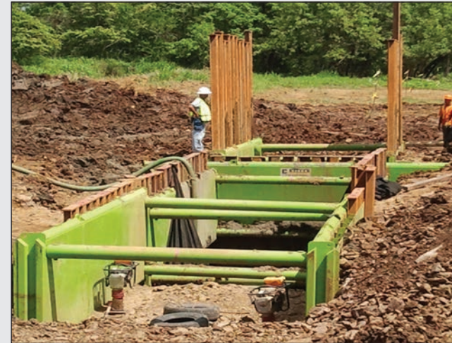
G3 System — 2 Sided application using spreader pipe.
